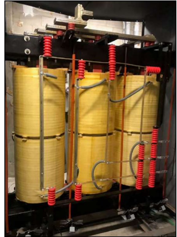
Successful Transformer Rebuild
