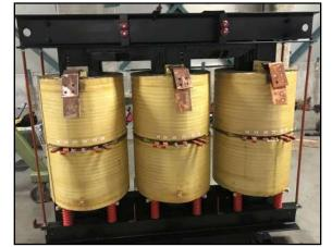
Top clamps and new insulators installed and then sprayed with dielectric varnish
